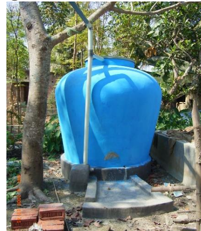
Dug Well Sand Filter (DWSF)
