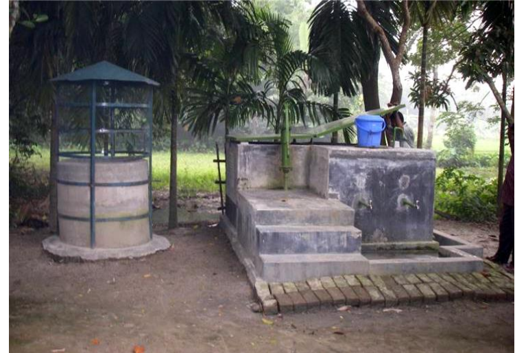
Dug Well Sand Filter (DWSF)
