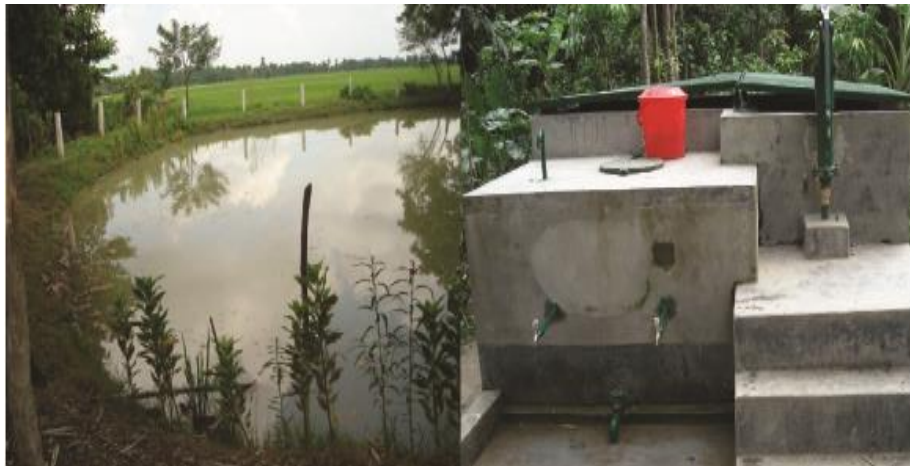
Pond Sand Filter (PSF)
