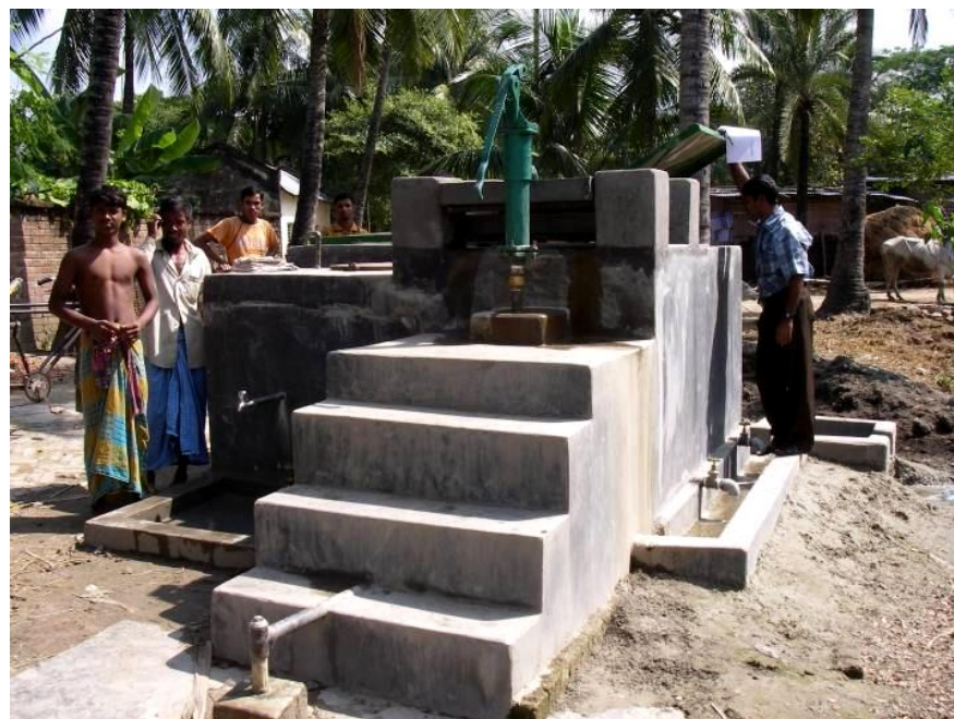
Arsenic Iron Removal Plant (AIRP)
