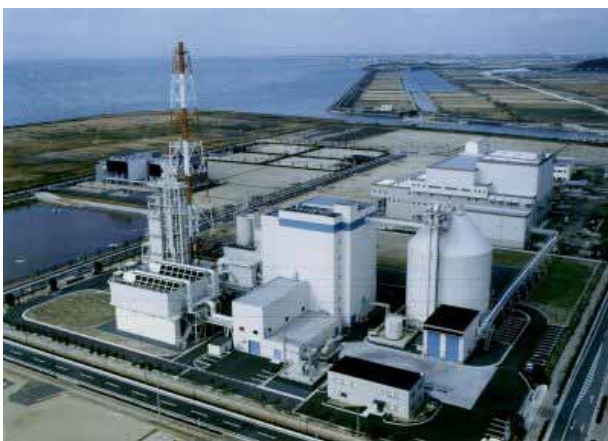
Photo: View of Omuta RDF-based Power Plant
