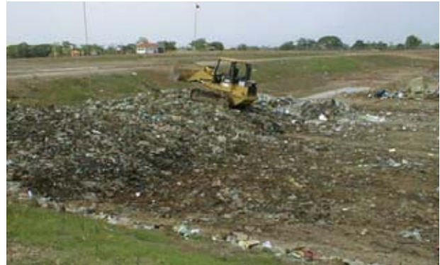
Waste Compaction at the Landfill using Heavy Machinery Granted by the Government of Japan
