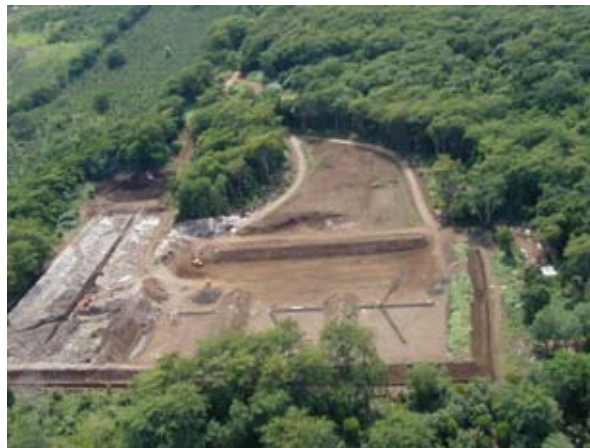
A big rubbish bin under rehabilitation
