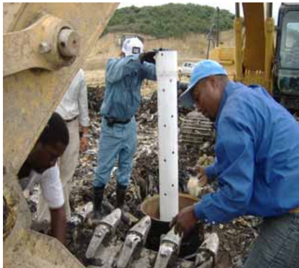
Instruction on installing the gas ventilation tube at the site
