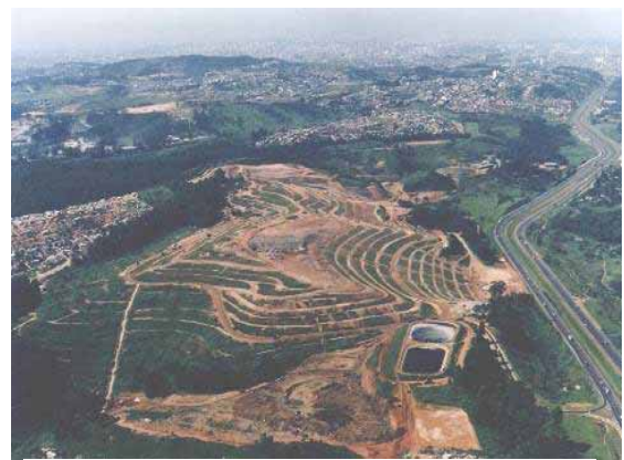
Picture 3.6: Power Generation Facility
