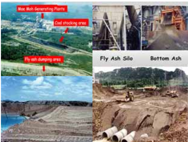
Photo2: Maemoh power station
