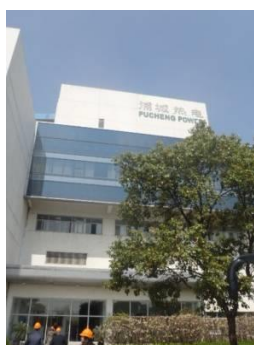
Entrance to the plant
