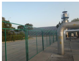
The black sheet on the slope at the back of the photo covers a completed landfill section
