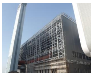
Under-construction Waste to Energy Plant
