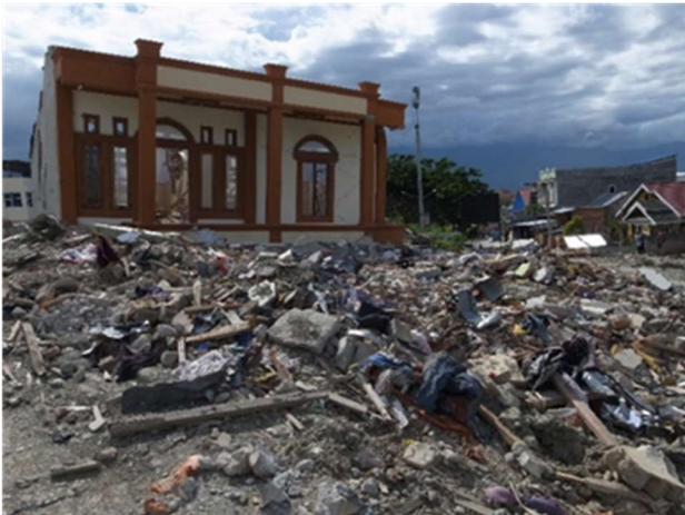
Damage from liquefaction and landslides in Palu City (Photo: Author)
