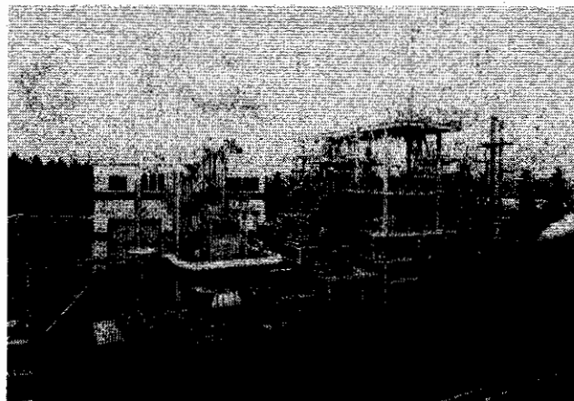
JWRF Plastics Waste Liquefaction Plant in Tachikawa
