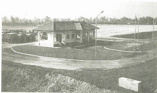
Completed KM18 Disposal Site
